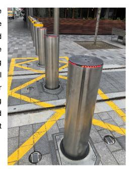
By placing static bollards on the perimeter, potential vehicle access has now been eliminated. These bollards act as a permanent protection barrier, stopping any vehicle from accessing the precinct. There are also benefits to installing static bollards in locations that require permanent protection at a perimeter. Static bollards allow for pedestrians to move about freely without compromising the protection against hostile vehicles or vehicles violating access.
