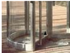
Framed toughened glass panels laminated 11.5mm thick with brush strips
