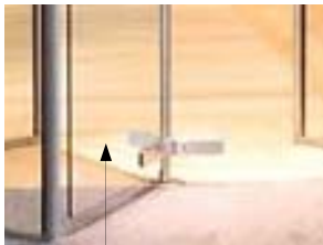
10mm thick toughened frameless safety glass
