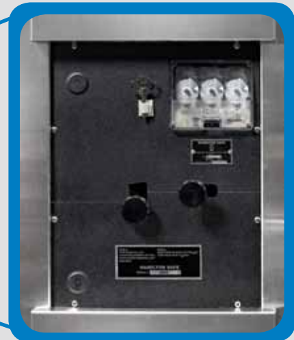
Emergency release built into door
